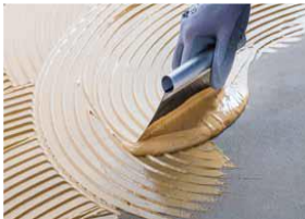
Picture 1. Trowel spread
